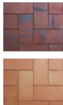
Clay Paving 200 x 100mm pavers laid on their sides, three colour variations used.
