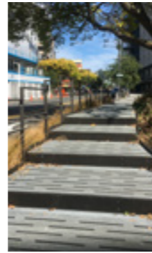
Rain Garden crossings. Slip resistant steel grating crossing over rain gardens.
