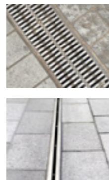
Surface Drainage. Drainage with removable grating for ease of maintenance.
