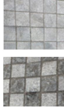
Stone setts. To define vehicle crossings on raised tables. (Potential to use existing setts in Council yard in pedestrian areas)
