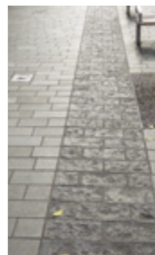
Tactile Band. 600mm tactile bands to define vehicle movement zone and for universal design purposes.
