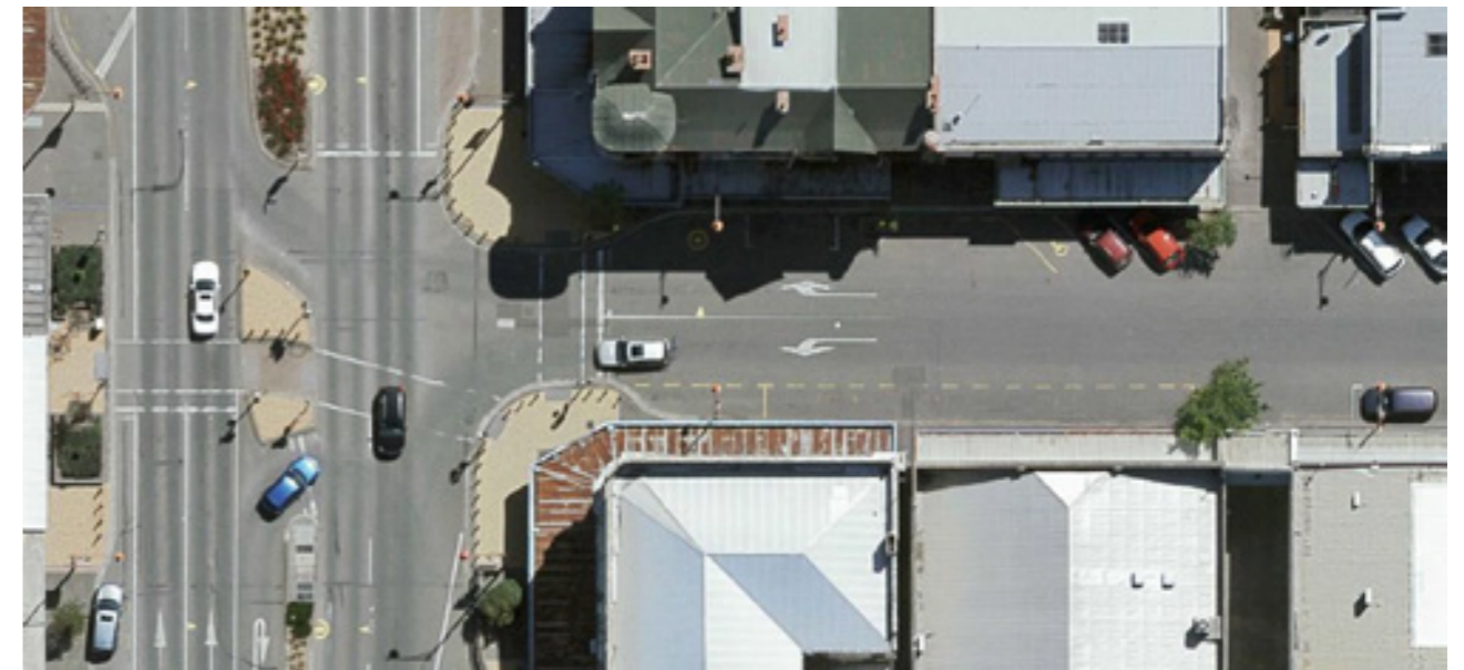
Figure 2.1 Existing Don Street intersection with Dee Street
